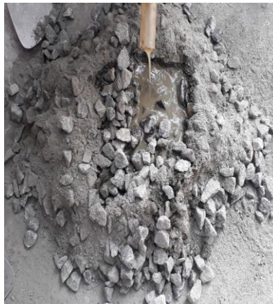
FIGURE 1. Casting of Concrete Specimens
